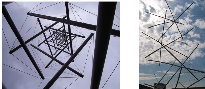
FIGURE 1. Examples of tensegrity towers. Left: Needle Tower II by Kenneth Snelson; Kröller-Müller Museum, Netherlands. Right: Photograph of a cane tower built by architecture students at the University of the Witwatersrand. 1
